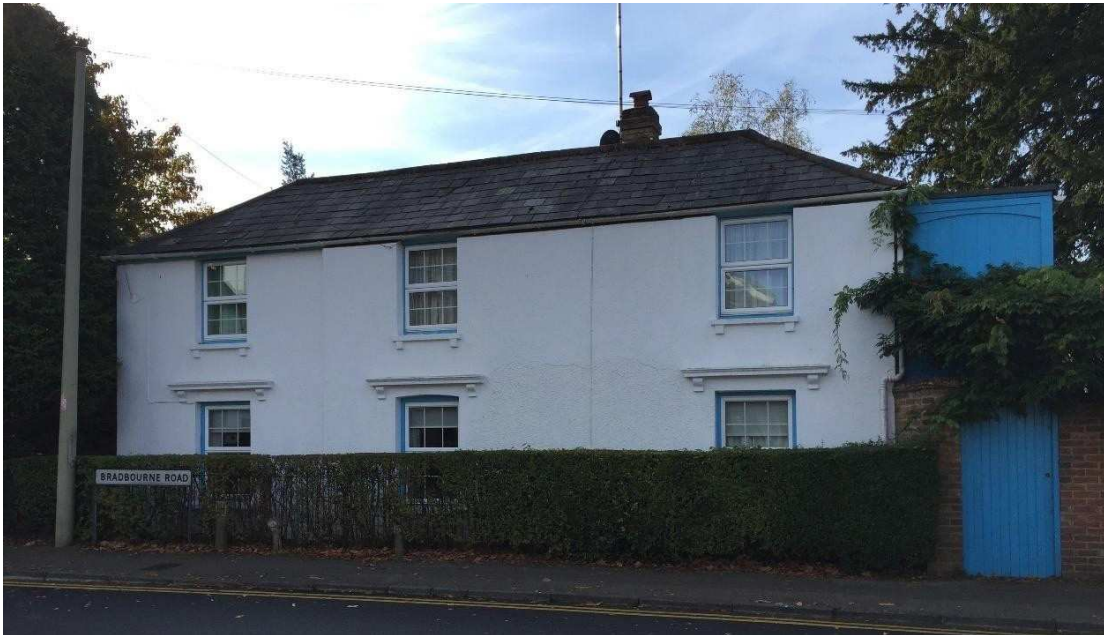
The Bradbourne Road elevation of 95 Dartford Road with replacement windows.
