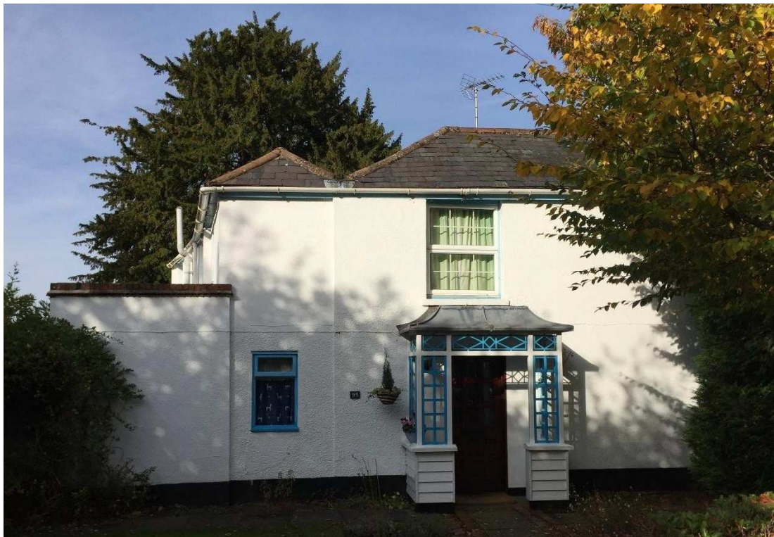
The Dartford Road elevation with modern porch structure and replacement windows.
