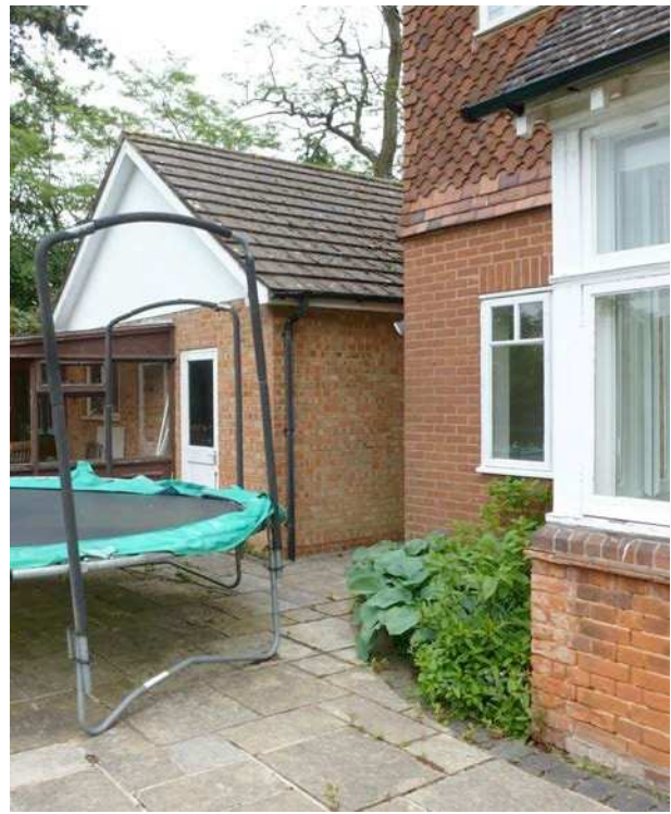
Above right: One of the double garages added either side of the house in the 1980's. To the rhs of the photo next to the bay window is the poorly matched brickwork of the 1970's staircase addition that was created to allow access to 1 st floor flat.
